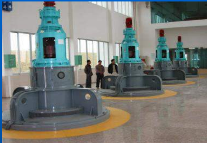
立式大型同步电机/ The large-scale vertical type synchronous motor
