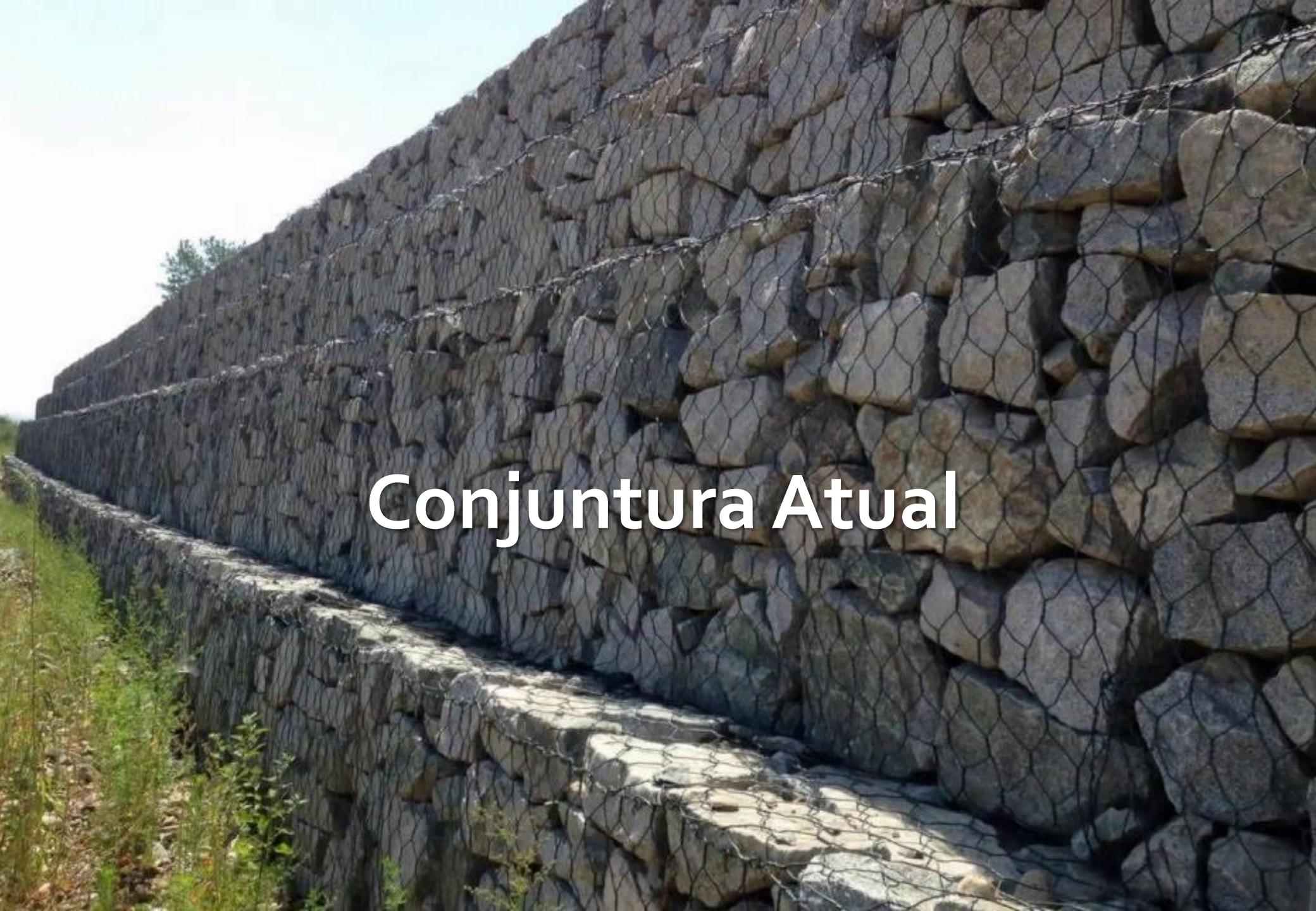
A photograph of a large-scale gabion wall. The wall is constructed from numerous rectangular stones stacked in a dry-stacked pattern, held together by a dense, black hexagonal mesh. The wall rises steeply from the bottom left towards the top right. In the foreground, there is a grassy embankment with some small green plants. The sky is clear and blue.
